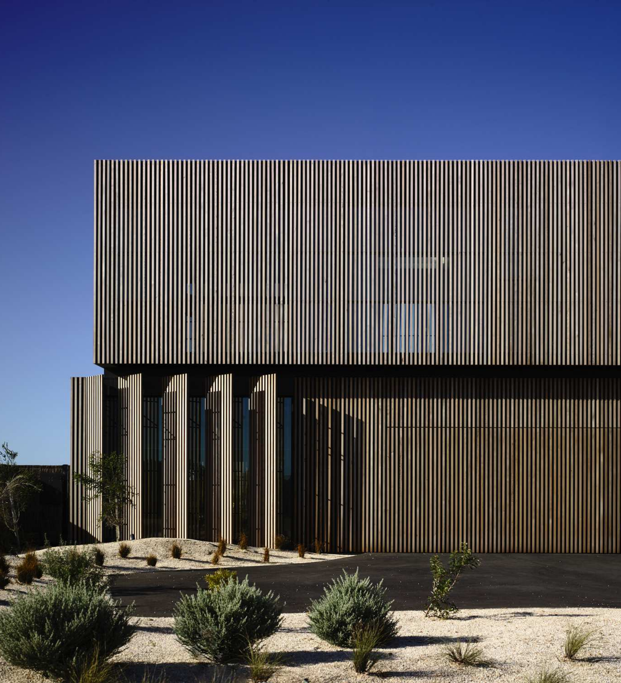
Stapeling van houten volumes in houten lamellen
